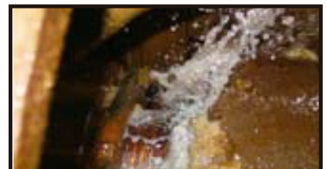
Gland packing 'slime out' consequences
