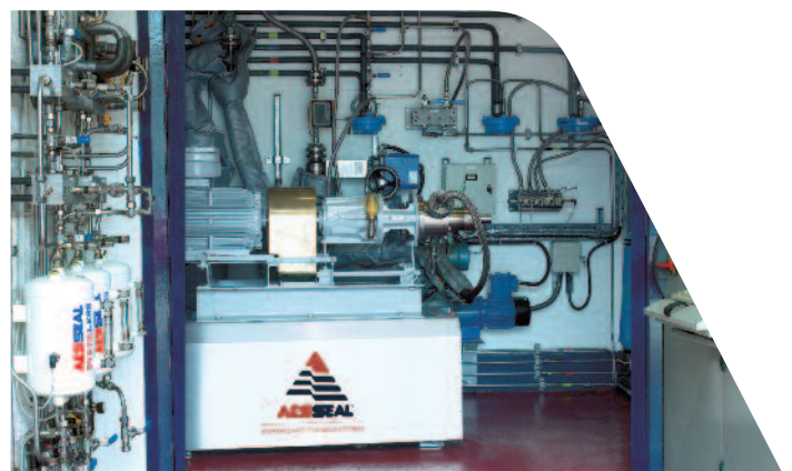
Extensive AESSEAL® test facilities
