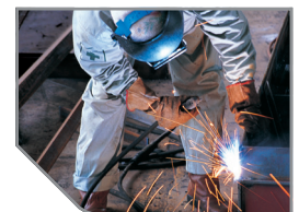
No torches / heat needed for repair
