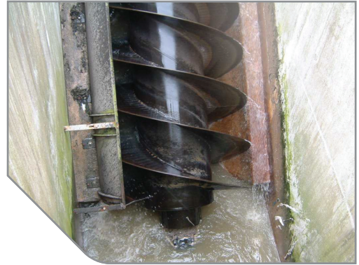
Archimedean screw fitted with AESSEAL® bearing seals in a UK sewage plant (Case Ref:1348)
